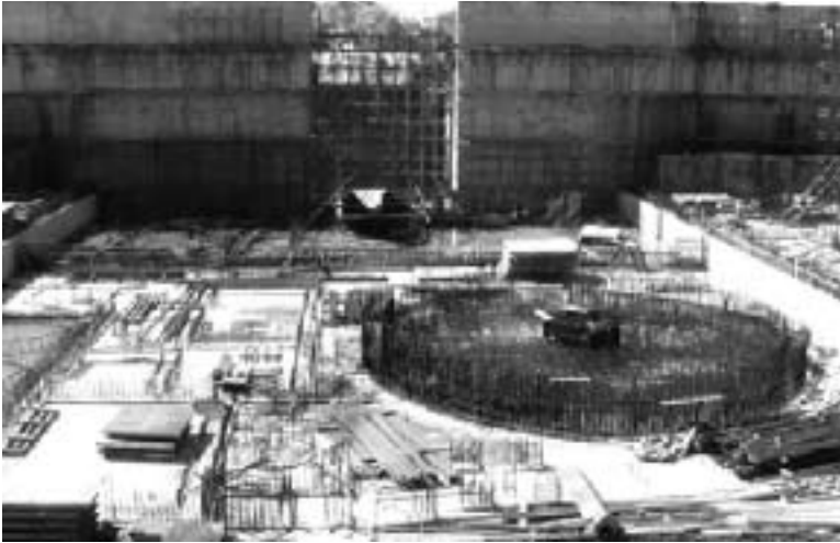
Figure 9. Construction Activity at Prototype Fast Breeder Reactor, Kalpakkam, April 2006. 103
