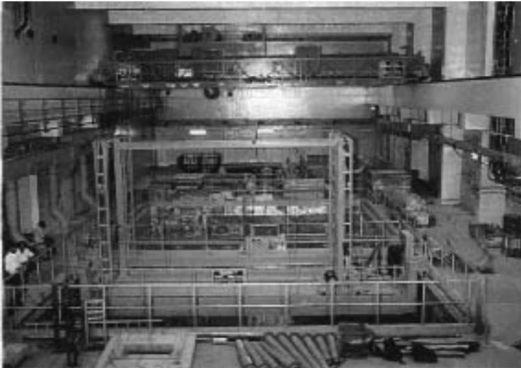
**Figure 4. Spent Fuel Pool and Fuel Handling Area, Kalpakkam Reprocessing Plant.**<sup>53</sup>
