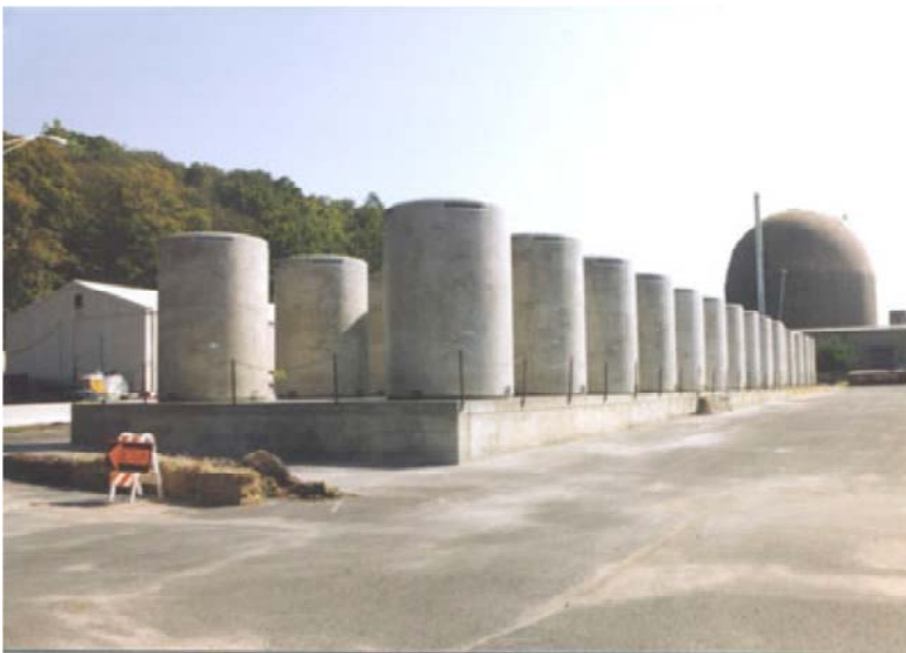
Figure 2. Dry-cask storage of older spent fuel at a U.S. nuclear power plant. Each cask weighs over one hundred tons and typically holds about ten tons of heavy metal (mostly uranium) in spent fuel that was discharged from the reactor twenty or more years earlier. A 1-GWe light-water reactor discharges about 20 tons per year. Each cask costs $1-2 million. Reprocessing of ten tons of spent fuel would cost on the order of $20 million. (Source: http://www.connyankee.com/html/fuel_storage1.html , accessed 16 December 2008).
